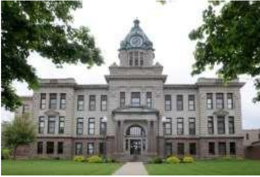
[Martin County Court House, Fairmont, Minnesota]
