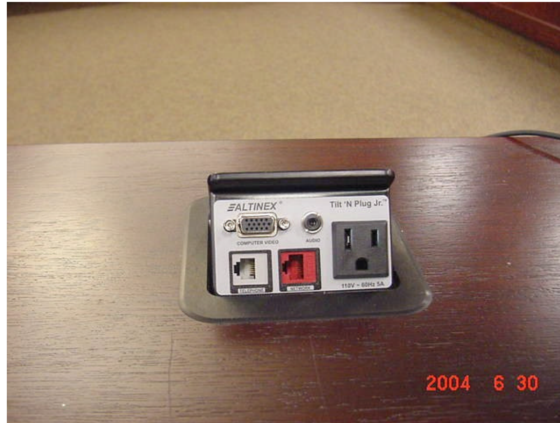
Fig 15: Pop-up connections on counsel table provide access to electricity, high speed Internet and telephone connections and computer input into the courtroom system.
