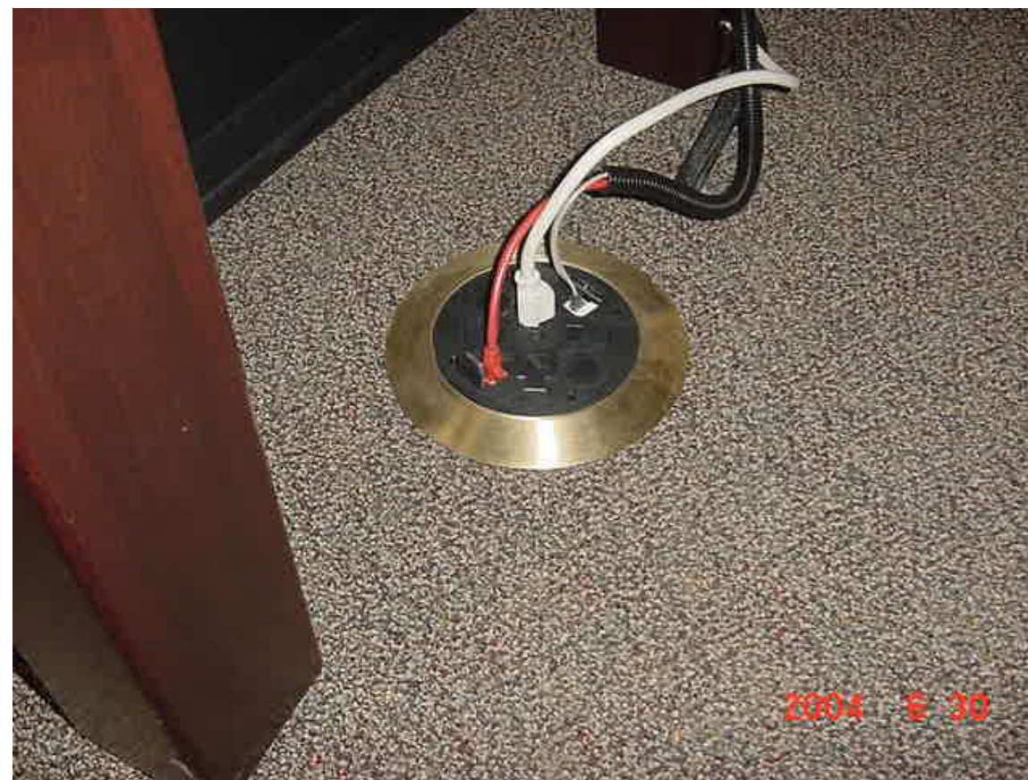
Fig. 13: The wiring for the counsel table pop-up connections runs through a hollow table leg to a floor hook-up.
