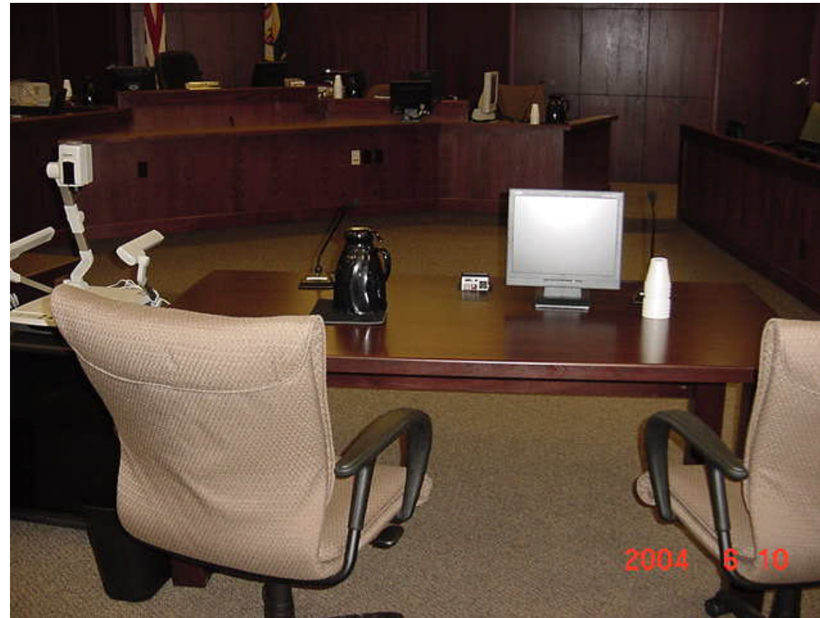
Fig. 14: Counsel table showing the proximity of the document camera and also the counsel table monitor. Note the direct line of sight to the witness.
