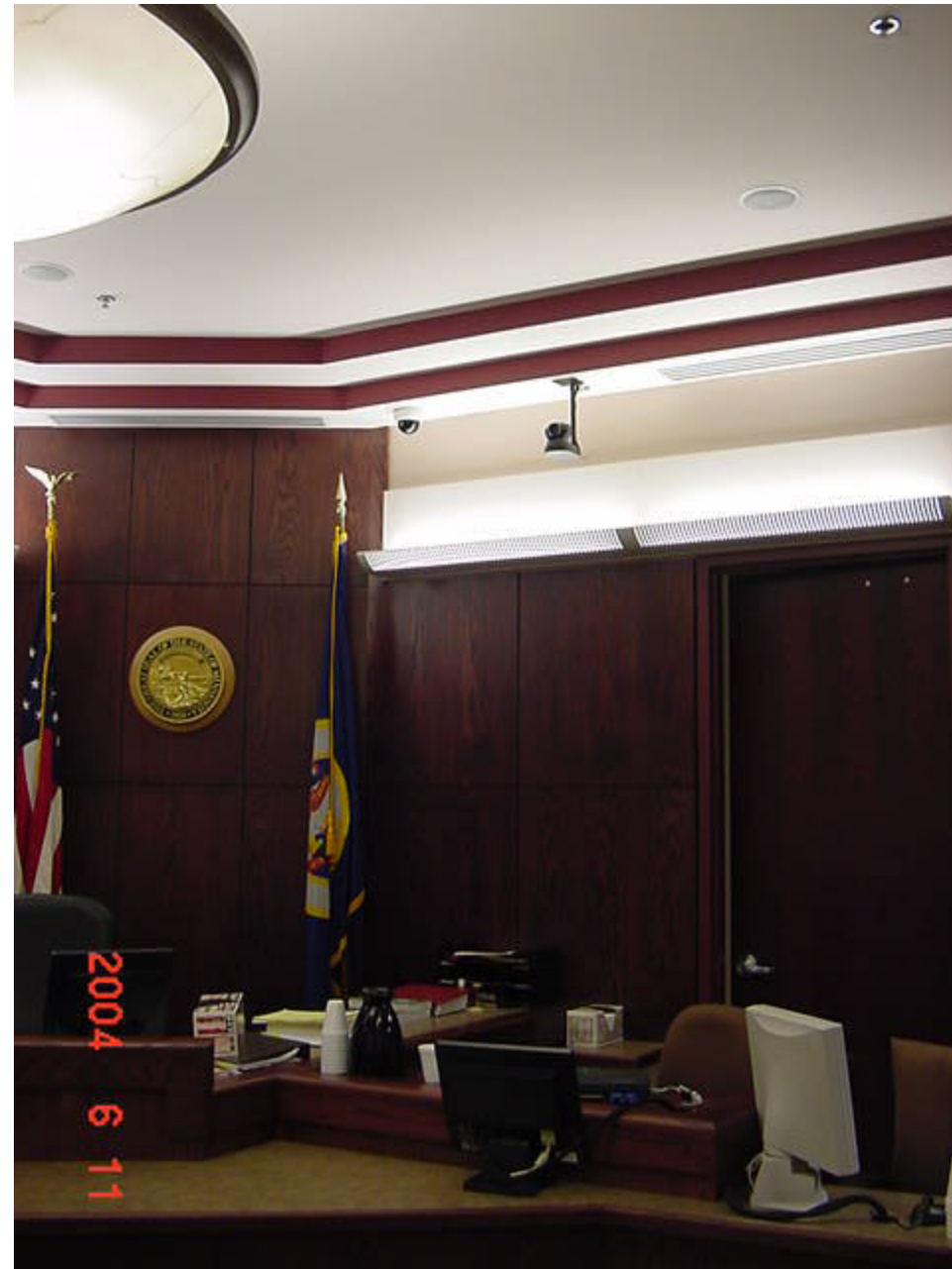
Fig. 25: View of one overhead camera for ITV. Compare its minimal intrusiveness with the large TV screens usually seen in courtrooms for ITV use. The lower part of the picture is a handy shelf in front of the Court and the court reporter for exhibits.
