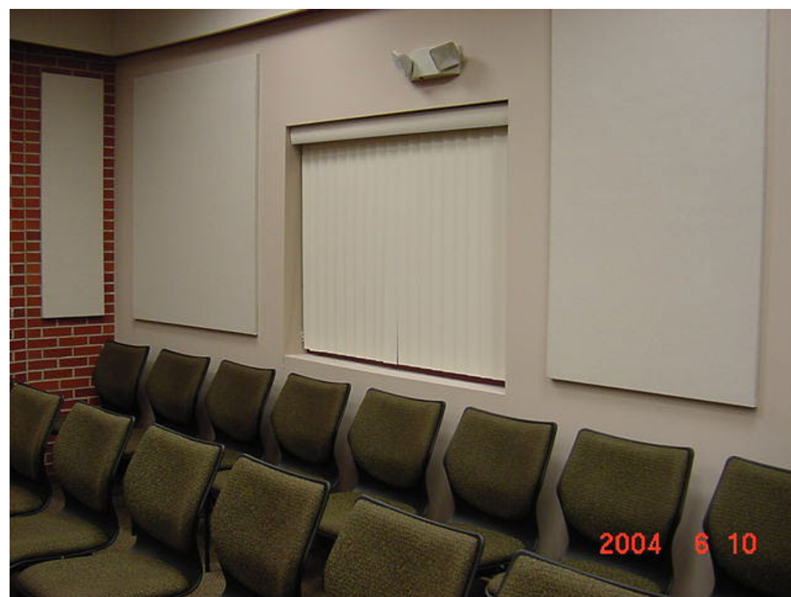
Fig.17: View of conference room window from courtroom with the blinds drawn for privacy.
