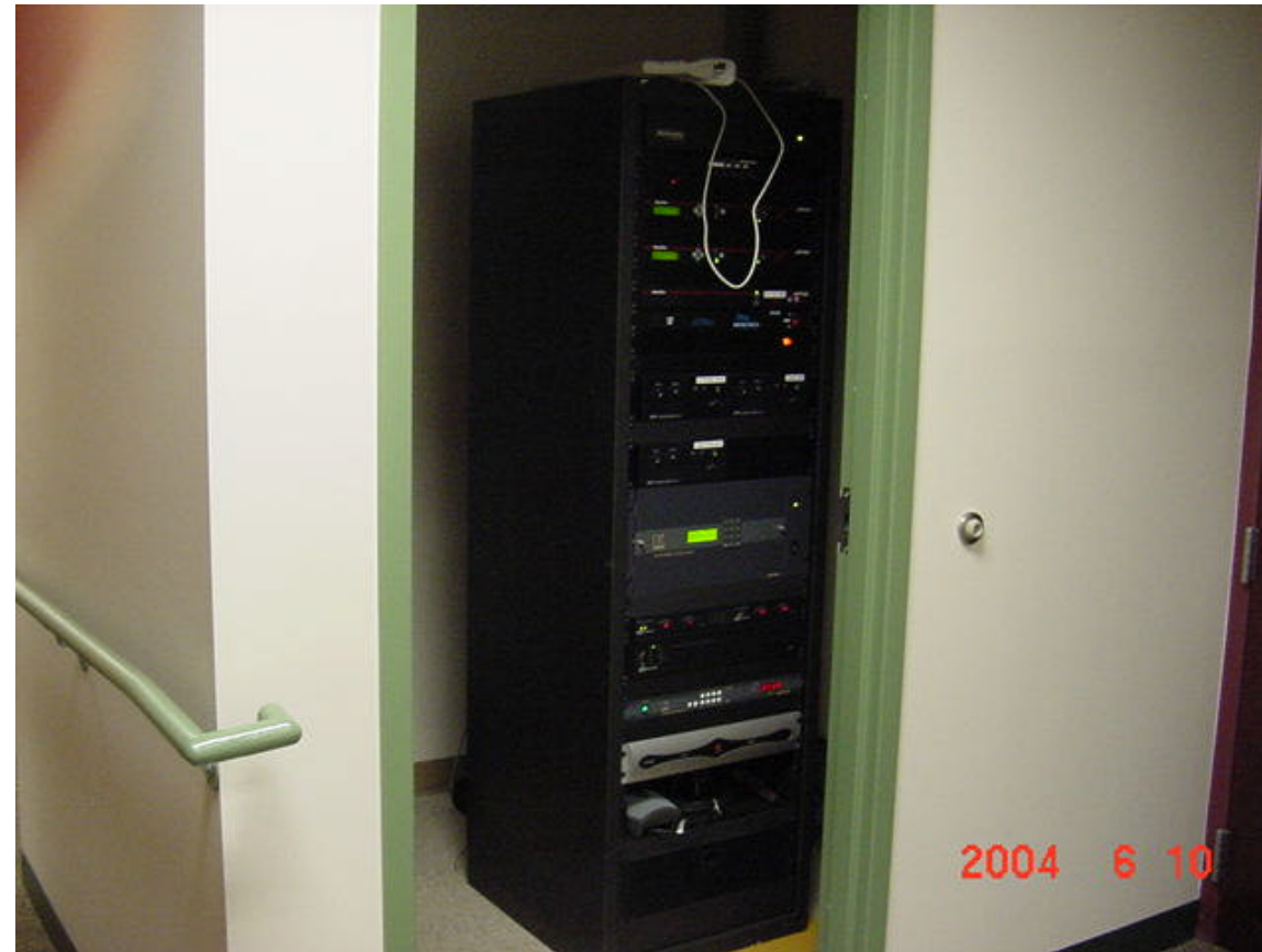
Fig. 2 - The rack is located in a closet behind the courtroom, accessible only to Court and staff.
