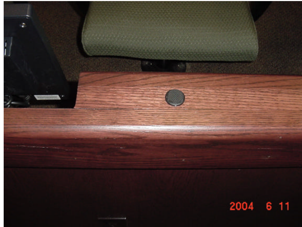
Fig. 12: One of seven button microphones on jury box rail.
