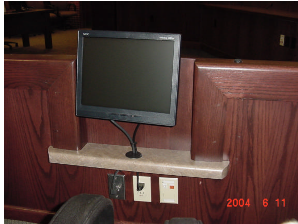
Fig. 13: Monitor in Jury box. Note that the monitors are protected from damage by jurors by being inset and the construction of a bumper shelf.
